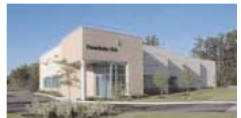
Building of CCL, CLT, and Fraunhofer USA Headquarters in Plymouth, Michigan
